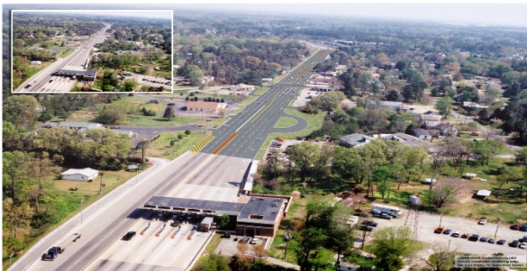
Above: The toll the end of the Colman Bridge, this is the southernmost point of 17 in Gloucester.
